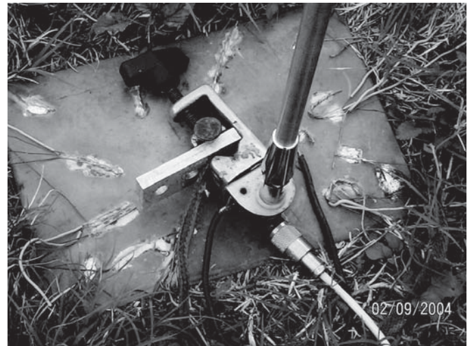
Figure 19 — Base mount over the radial system.
